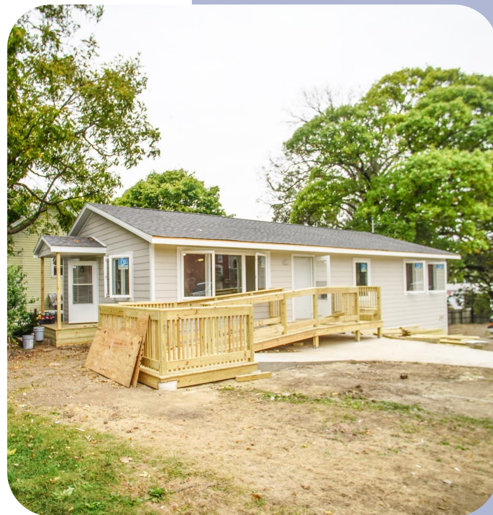
Home Repair & Accessibility Program, Bloomington
